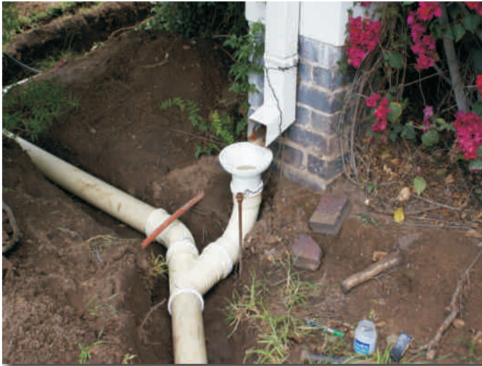
Rainwater from the extensive clay-tile roof is collected through downpipes of the gutters and...
