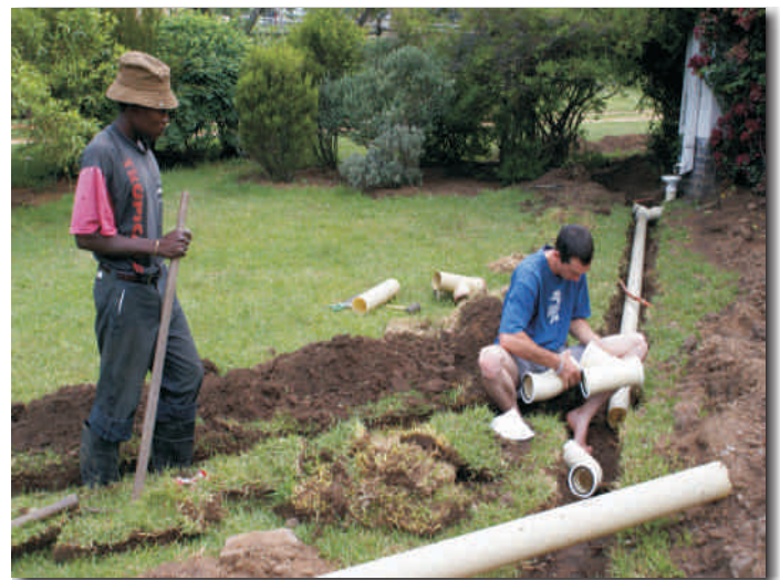
... and fed through a specially designed filtering trough which is also a plant-bed, from where it flows through drainage pipes into the pool to be used for irrigation and fish-farming.
