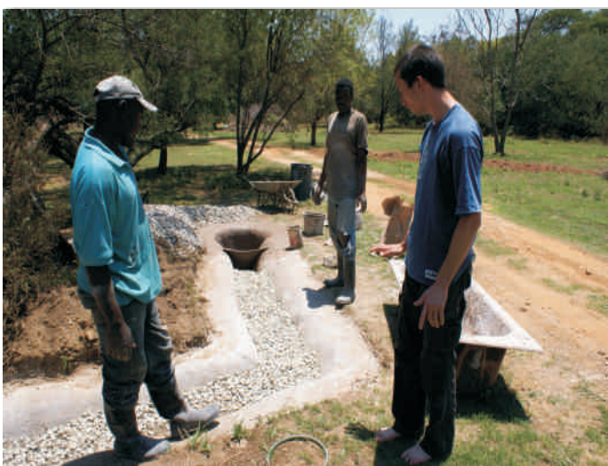
In both these images, grey water is captured from the dwellings' bathrooms and kitchens and channelled through specially built canals, feeding plants with recycled municipal water.
