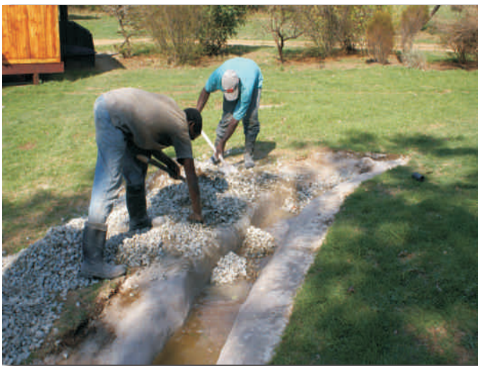
... and fed through a specially designed filtering trough which is also a plant-bed, from where it flows through drainage pipes into the pool to be used for irrigation and fish-farming.
