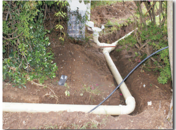
Rainwater from the extensive clay-tile roof is collected through downpipes of the gutters and...
